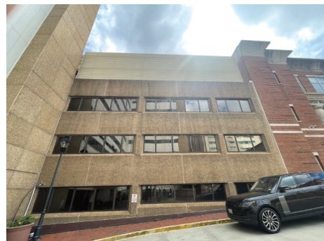
VIEW OF EXISTING PRECAST CONCRETE PANELS
