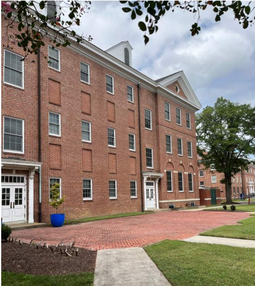
East Elevation, standing from the path
