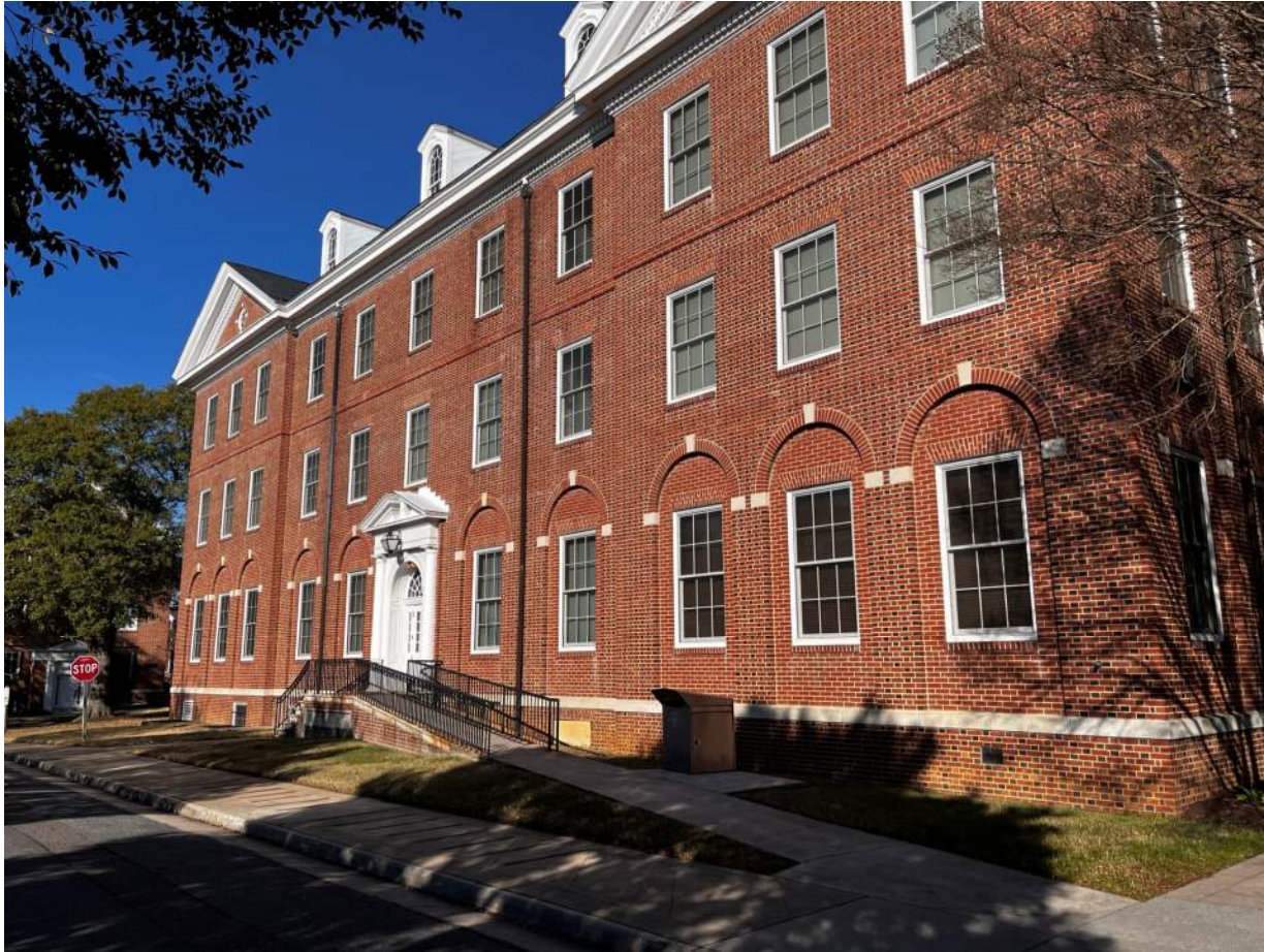
West Elevation, looking from Hayden Drive near south end of building
