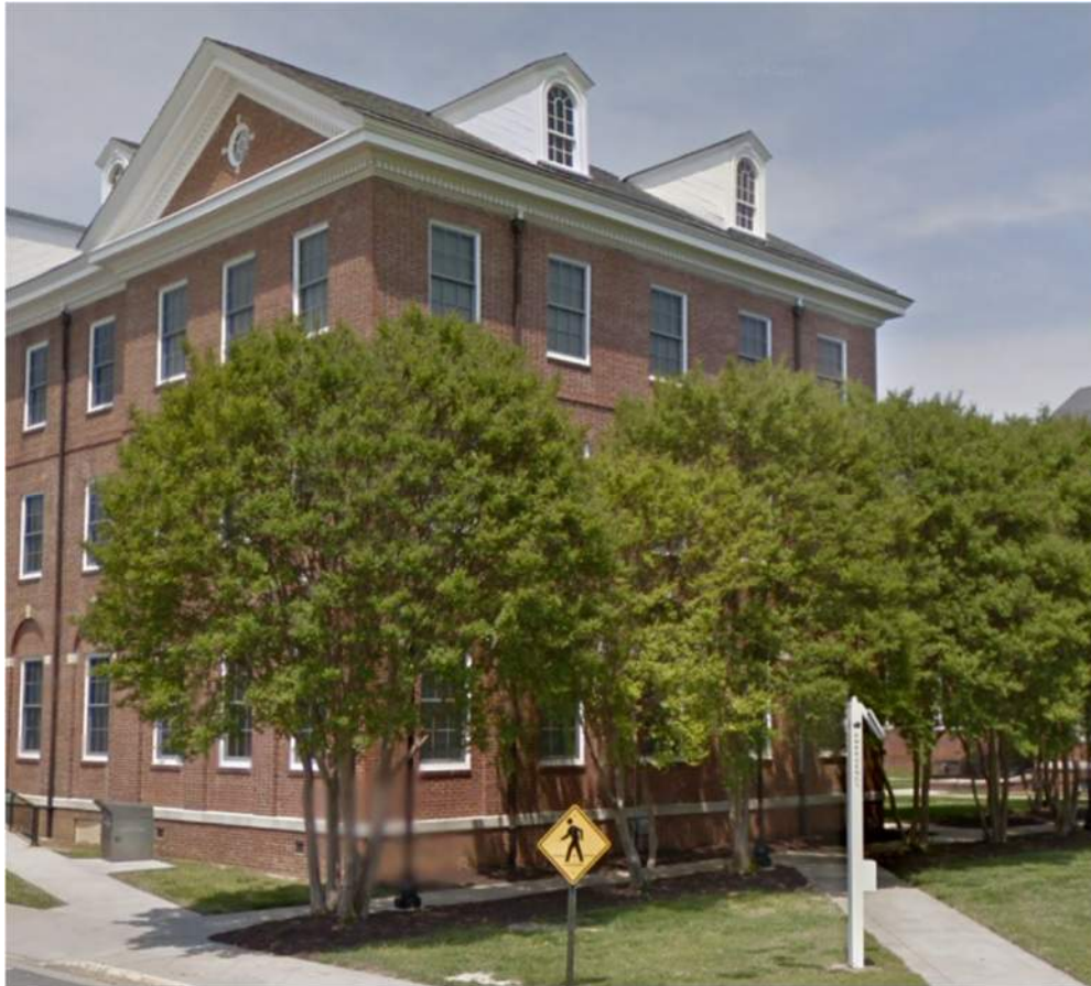
South Elevation, looking from Hayden Drive
