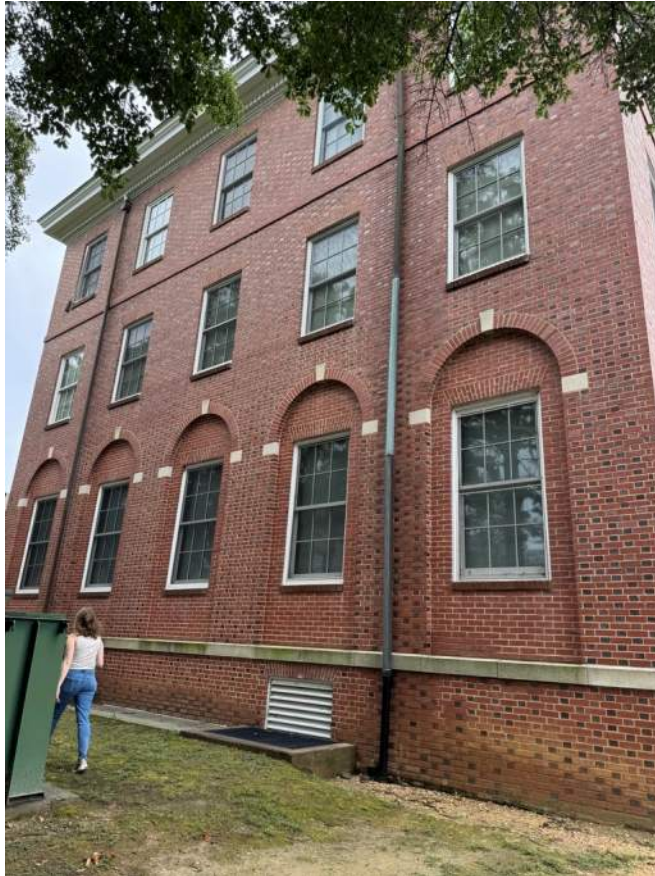
North Elevation, side of building near corner of Hayden Drive and Hayden Street
