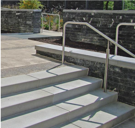
Precast Stair and Wall Cap and Stainless Railings
